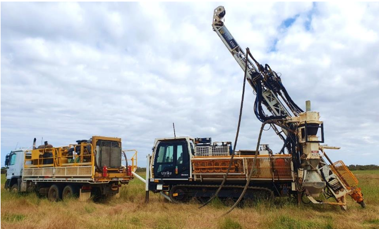
Figure 5: Drilling at Springdale
